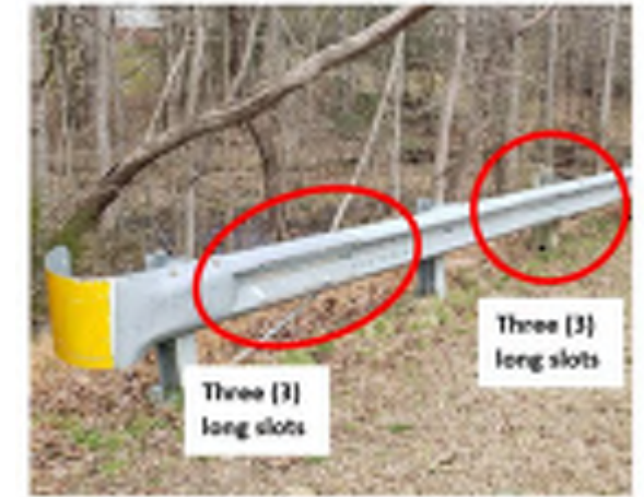
Six (6) long slots seen on Trinity SRT-350 GR-7 Terminal
