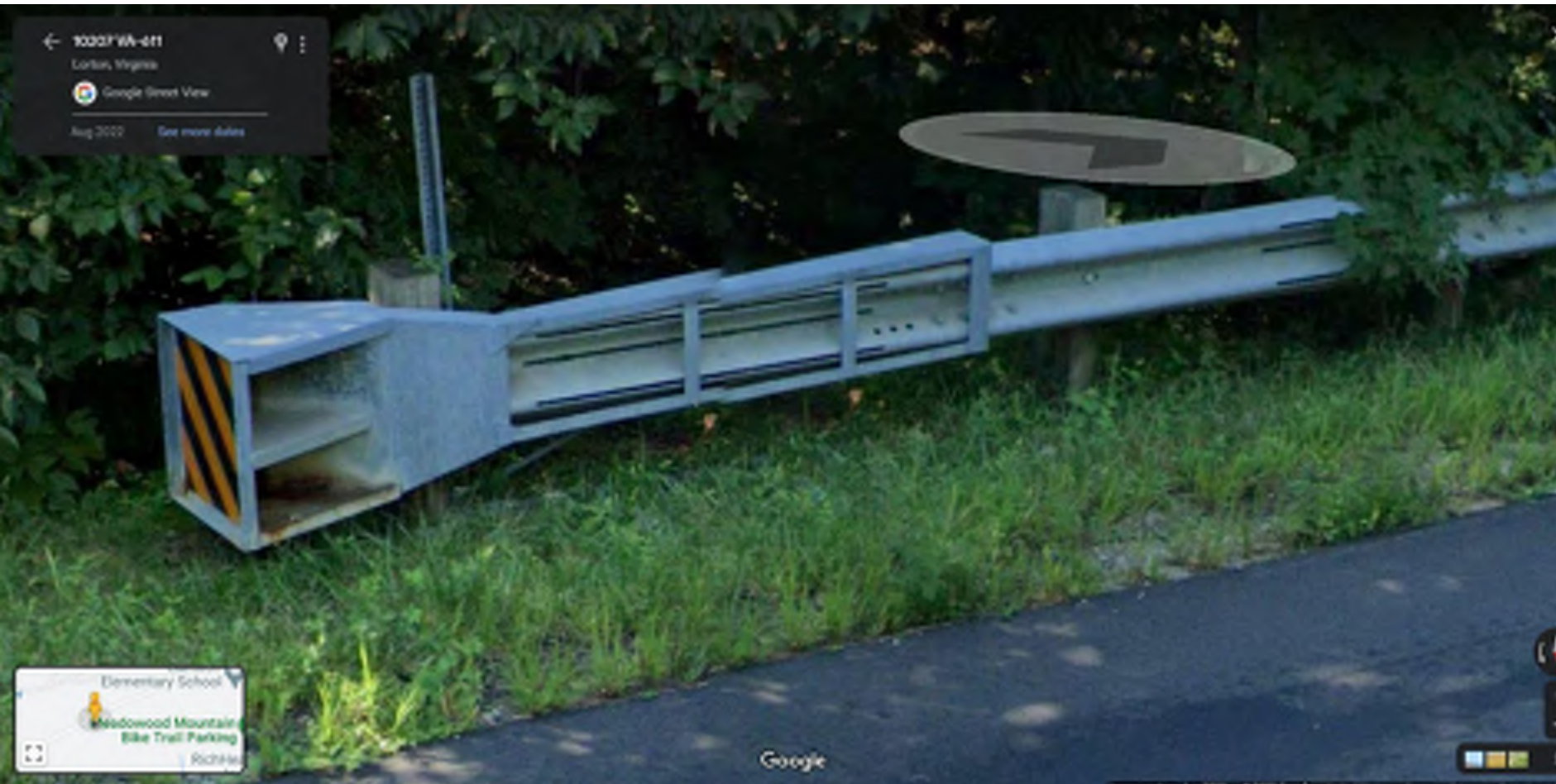
Three (3) short slots seen on Road Systems SKT-350 GR-9 Terminal (front)
