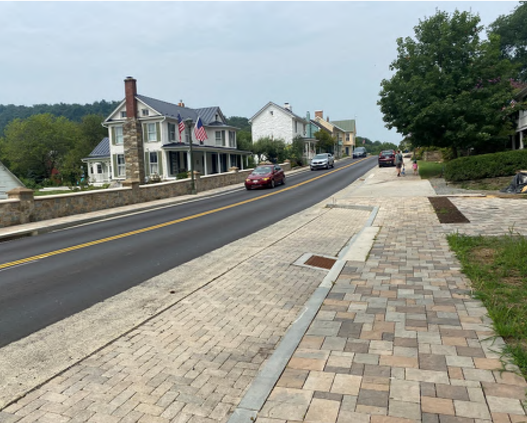
Create a Complete Street with a narrower roadway, new curb and gutter, parking lane, and sidewalks on both sides.
