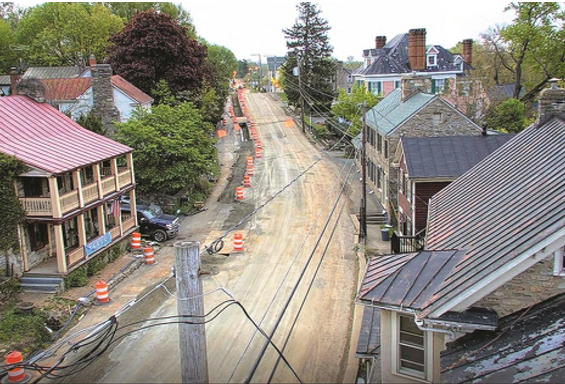
Asphalt roadway one side to the other.
